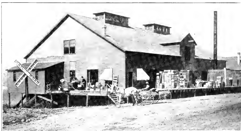
Lewiston-Clarkston Canning Co.'s Plant, Lewiston, Idaho
